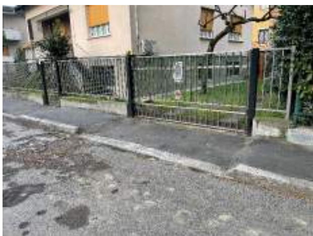
B1.7 rampe non adeguate
